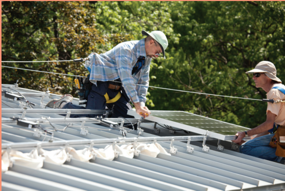
A PV solar array was installed on the upper roof by Re Power Solutions.
