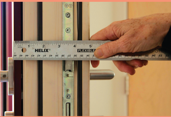
Thick, vaultlike doors with multipoint locks and latches.
