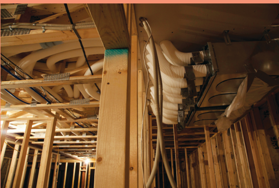
The only ductwork in the house was for fresh air intake and stale air exhaust (4-inch ERV ducts).
